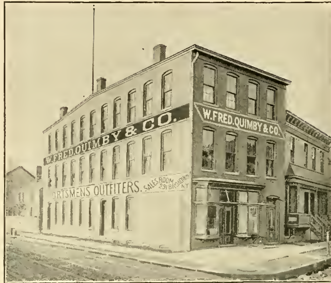
W. FRED QUIMBY CO., PENN. R. R. AVENUE CORNER SOUTH STREET.
